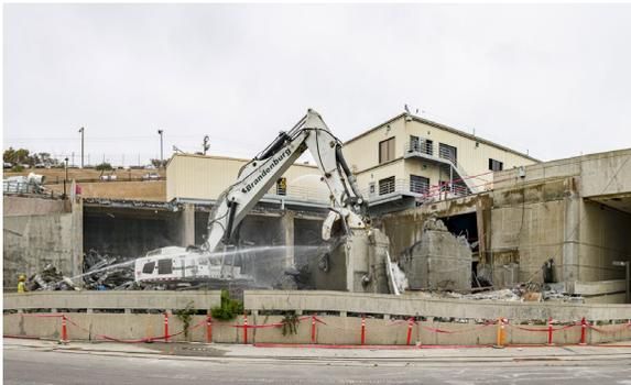
*Spraying water during demolition is one technique for controlling dust and debris while the main office building is being dismantled.*
