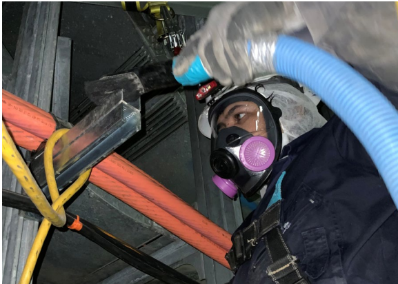
Trained worker removes asbestos from Containment
