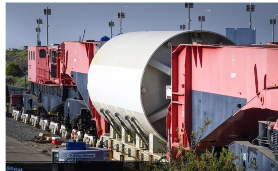
After being stored on site for more than 20 years, the Unit 1 reactor pressure vessel was shipped in May to the EnergySolutions facility in Clive, Utah for final disposal.
