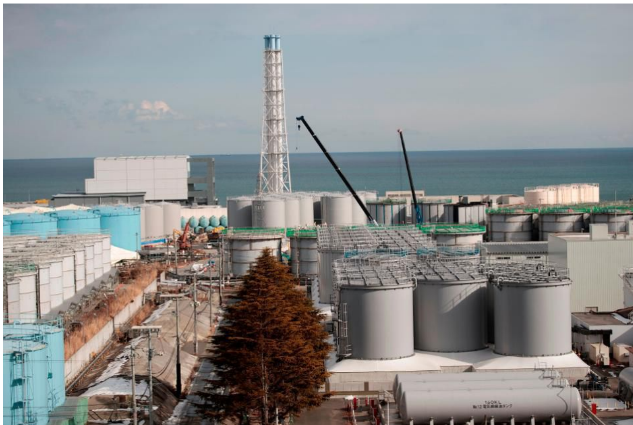
A reactor building and storage tanks for contaminated water at the Tokyo Electric Power Company Fukushima Dai- [ + ]
