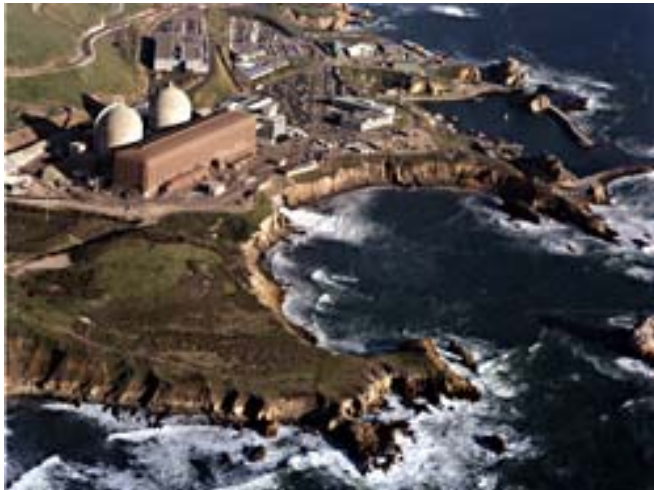
Diablo Canyon Power Plant
