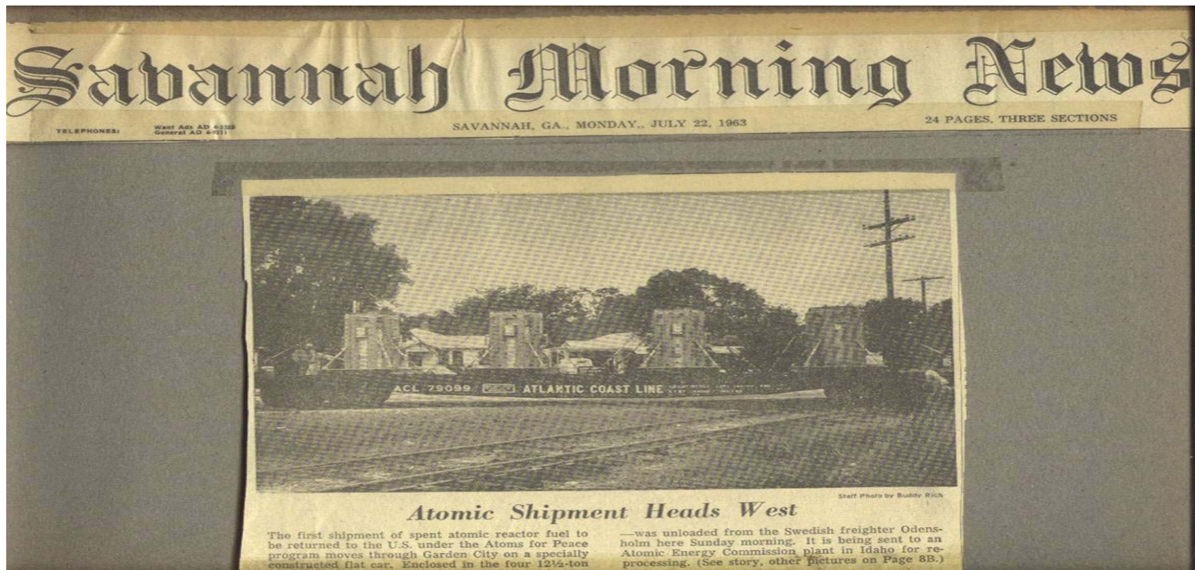
First Shipment of Spent Reactor Fuel in 1963
