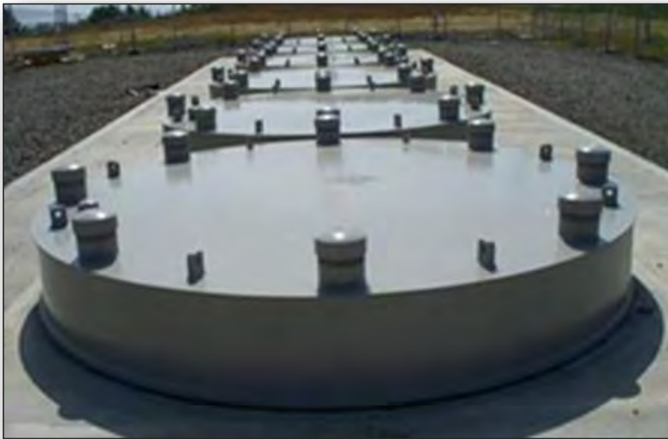
Underground Vertical Dry Storage Systems at Humboldt Bay (2006)
