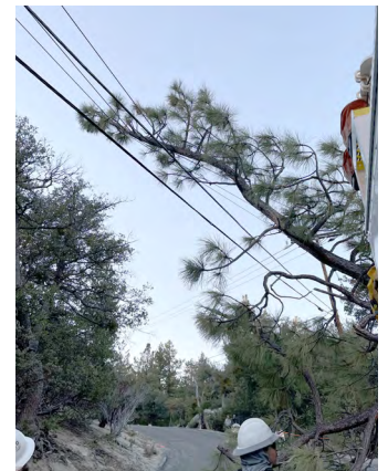
Inspection photos show tree branches that came into contact with wires featuring the protective coating (covered conductor). Power remained safely on for customers in the Idyllwild area of Riverside County - Nov. 25, 2021. Credit: Trenton Koury
