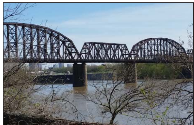
K&I Railroad Bridge
