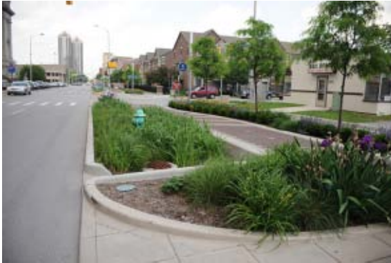
Figure 5-10 Bioinfiltration is an example of a source control structural solution
