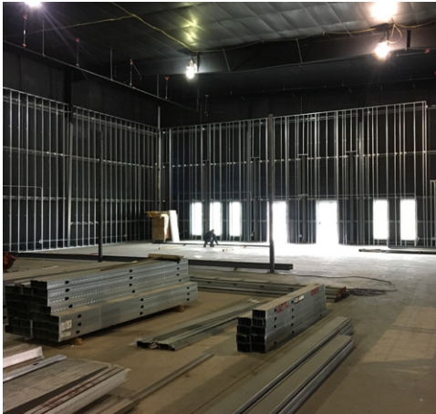
Progress continues at the building site!
