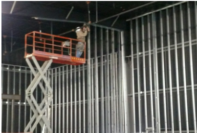
Working on the walls
