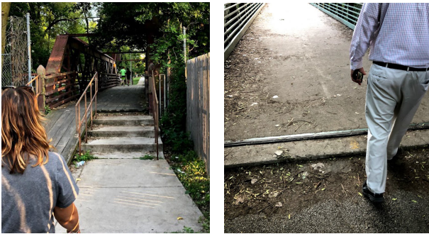
Image: Thresholds at bridges are not ADA or bike friendly
