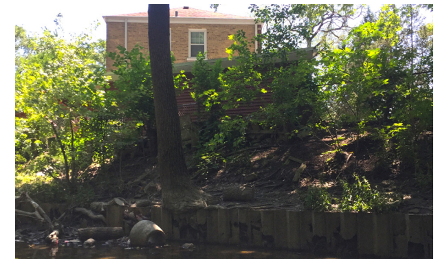
Image: Decayed sheet piling / seawall on private property
