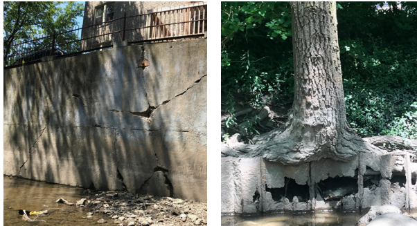
Image: Decaying concrete and sheet metal retaining walls
