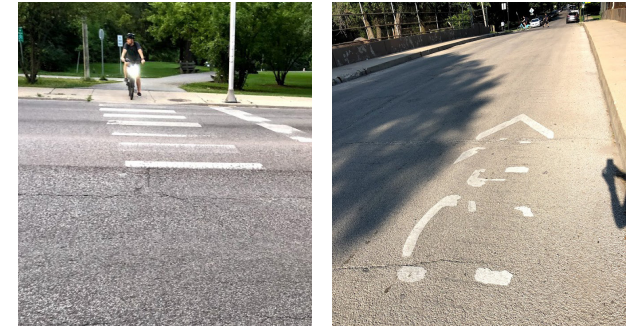
Image: Example striping and bike markings that need repainting
