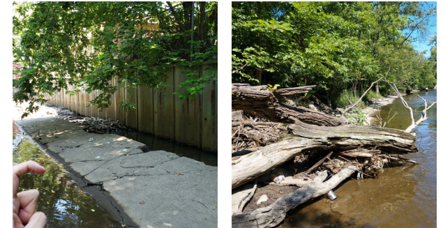
Image: Example of exposed concrete liner, and log dam
