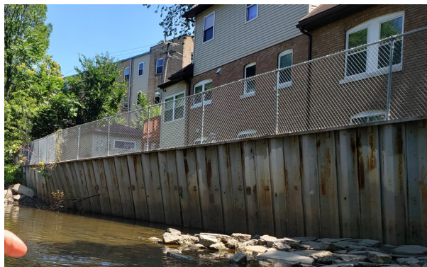
Image: Failing retaining wall on private property
