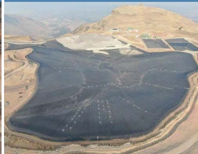
Heap Leach Pads 1A and 1B
