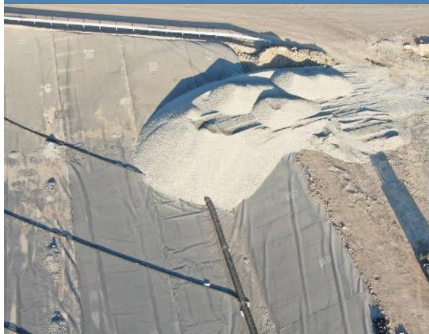
Heap Leach Pad 1A+1B Overliner
