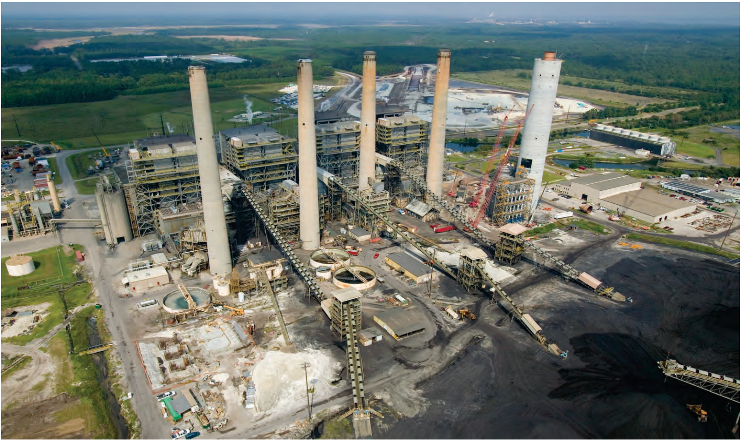
Santee Cooper Winyah Generating Station located in Georgetown, SC.
