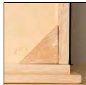
All drawers are constructed with 4 corner blocks
