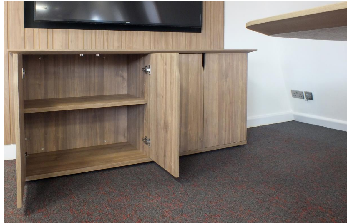
Soft close hinges, internal adjustable shelf.
