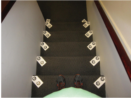
Top of Stairs, No Landings
