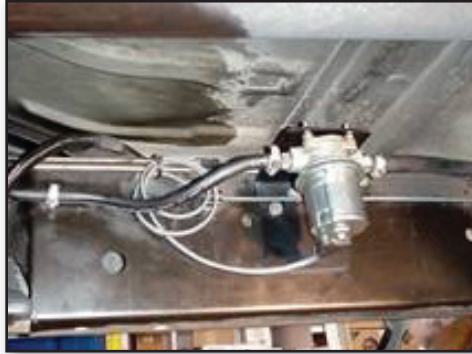
The finished installation.
