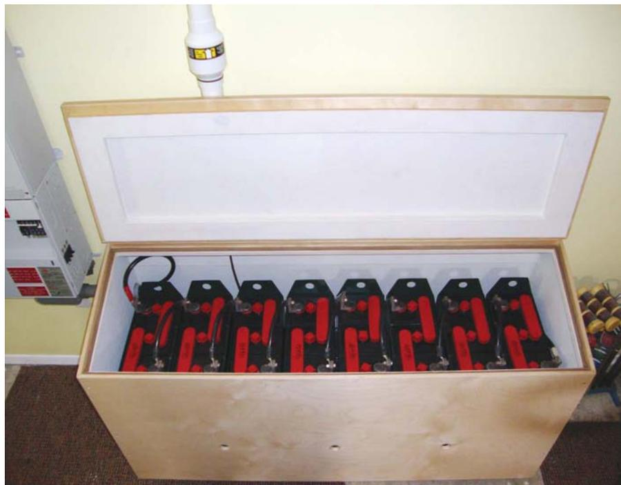
To secure battery conduit fittings to the battery box, we use two concentric hole saws from opposite sides, creating a 1/4-inch-thick flange to fit a lock ring around 1 1/2-inch (for 2/0 cables) or 2-inch (for 4/0 cables) battery conduit. This allows the threads of the conduit fitting to get into the box
