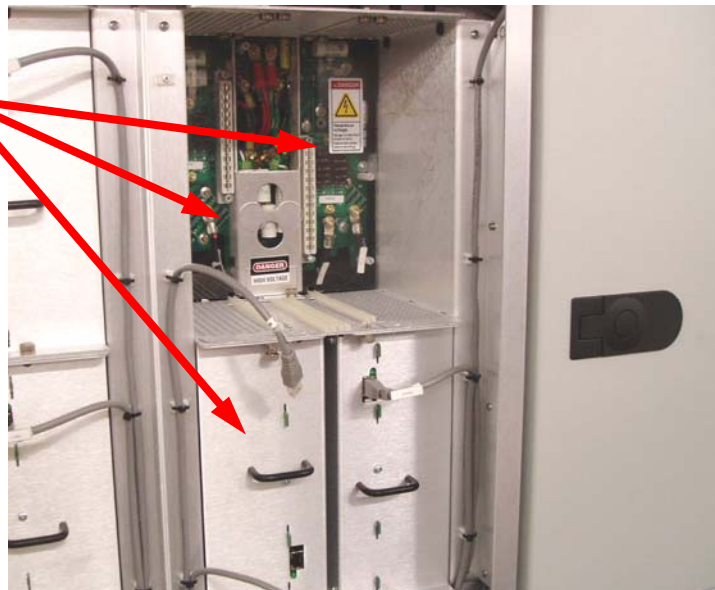
Figure 22 – Install PA Modules
