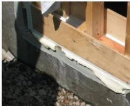
5. Caulk inside and out along joint between Premier Window and wall. TapCon screws (1-2) into jambs to secure window.
