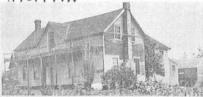
The Folly House built in 1800. Photograph courtesy Library of Congress
