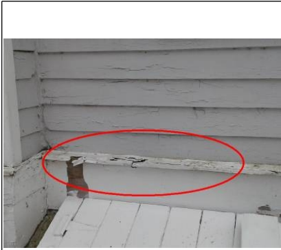
Moisture damage to wood
