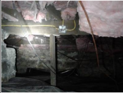
Post support installed
