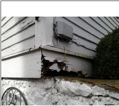
Moisture damage to wood
