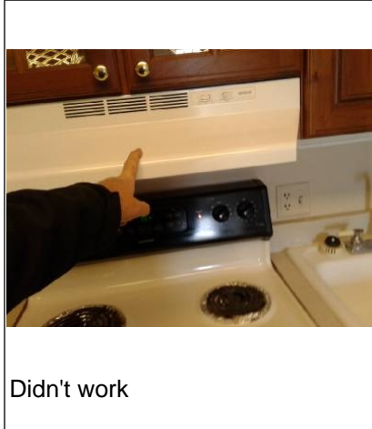
Open ground and not GFCI protected
