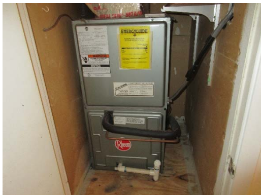
Electric Heating Unit – 2002 – 3 Ton
