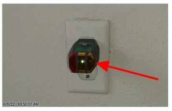
The living room has an ungrounded 3-Prong outlet on the west wall that needs service by a professional in the electrical field.
