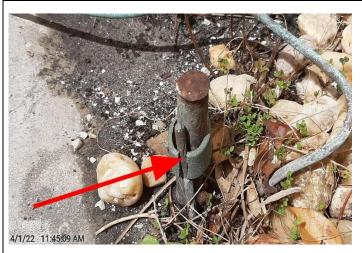
Ground clamp is loose or damaged at ground rod that service is needed by a professional in the electrical field.
