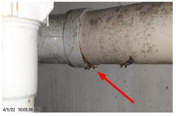
The PVC waste drain pipe in the garage is leaking and needs service by a professional in the plumbing field.
