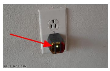
The dining room has an ungrounded 3-Prong outlet on the east wall that needs service by a professional in the electrical field.
