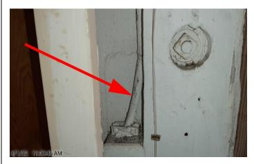
There is exposed wiring in the garage on the front wall that should be in conduit or covered and needs service by a professional in the electrical field.
