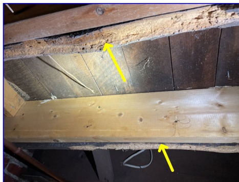
Powder post beetle damage
