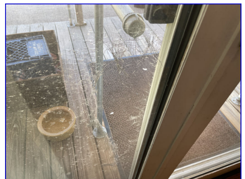
Damaged screen
