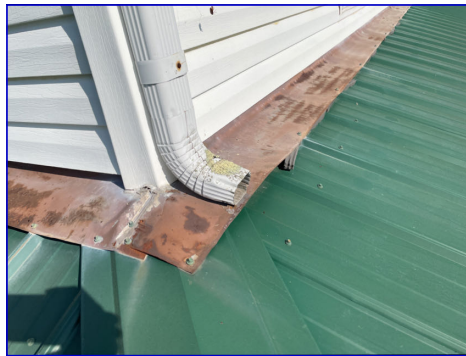
The flashing is rusting. It should be painted to extend its life.
