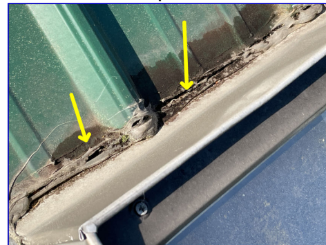
The skylight flashing is vulnerable and should be carefully monitored for leaks.(heavy sealant usage)
