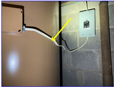
Wiring serving the electric water heater should be protected by a conduit.
