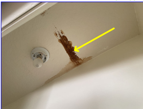
An apparent water staining was noted (East bedroom).
