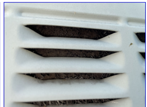
The outdoor unit of the air conditioning system requires cleaning.
