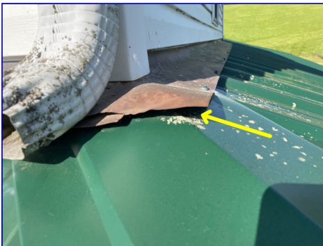
The flashing is loose and should be re-secured to avoid leaks.
