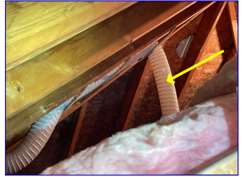
Consider wrapping shower vent duct in insulation to help prevent condensation forming in extreme cold temperatures.
