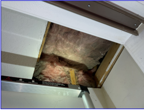
Attic hatch cover was missing.
