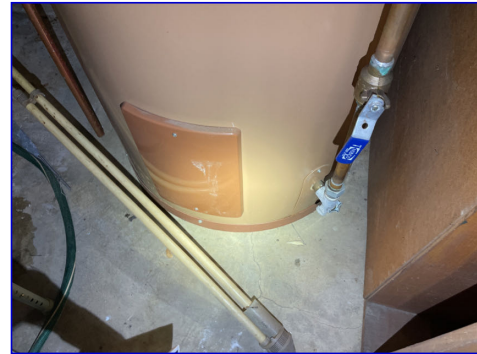
No signs of leaking at water heater
