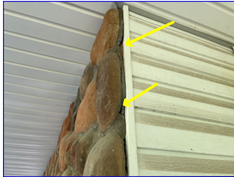
The siding is lacking proper sealant joints at intersections (Stone meets trim intersections, etc.)
