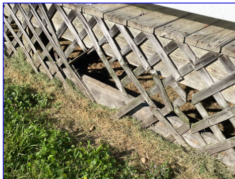
The lattice is damaged. It should be replaced.
