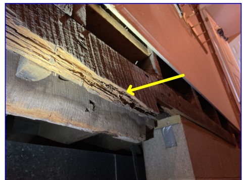
Termite damage
