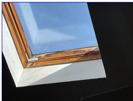
Water staining was observed around the skylight windows. No active leaking found. Monitor.
