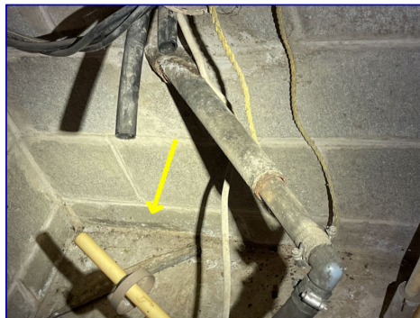
The basement shows evidence of common moisture penetration.
