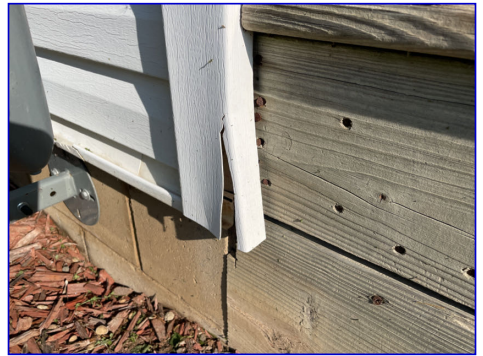
The siding is damaged at (south) and should be repaired or replaced.
