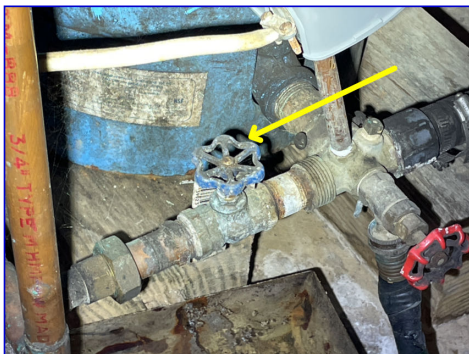
Main water shut off valve
