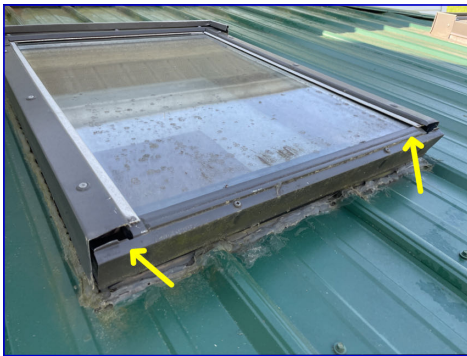
The flashing is damaged and should be repaired to avoid leaks.
