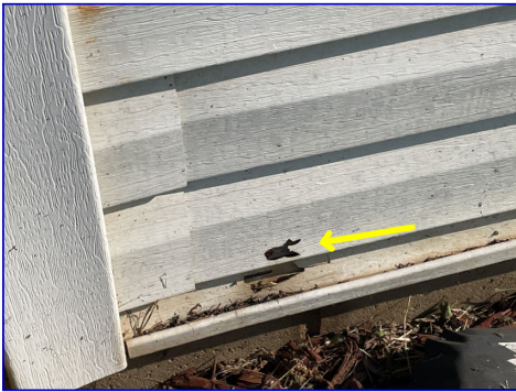
The siding is damaged at (south) and should be repaired or replaced.
