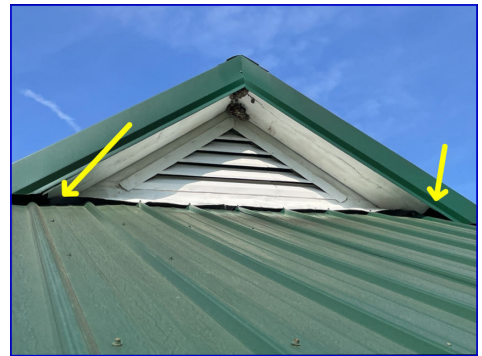
The installation of the flashing is incomplete and should be repaired to avoid leaks.
