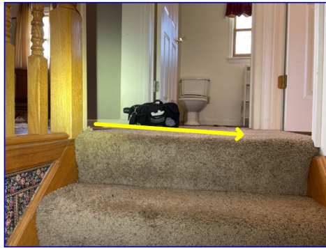
Floor slopes are apparent.
