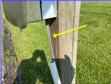
Wiring exposed on exterior should be protected by a rigid conduit (near driveway).
