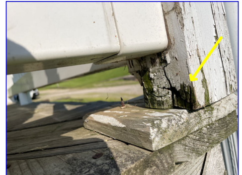
One porch post base is dilapidated. It should be replaced.
