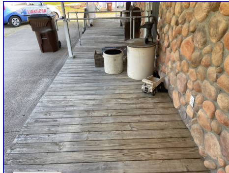
The deck should be painted or stained to improve durability.
