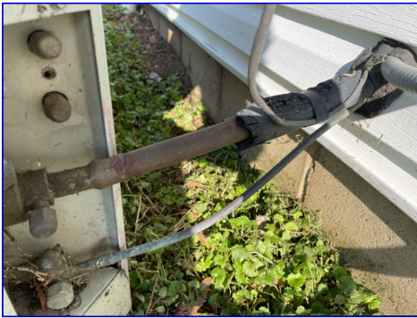
Damaged and or missing insulation on refrigerant lines should be repaired.
