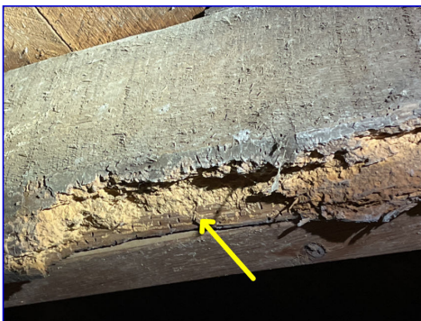
Powder post beetle damage
