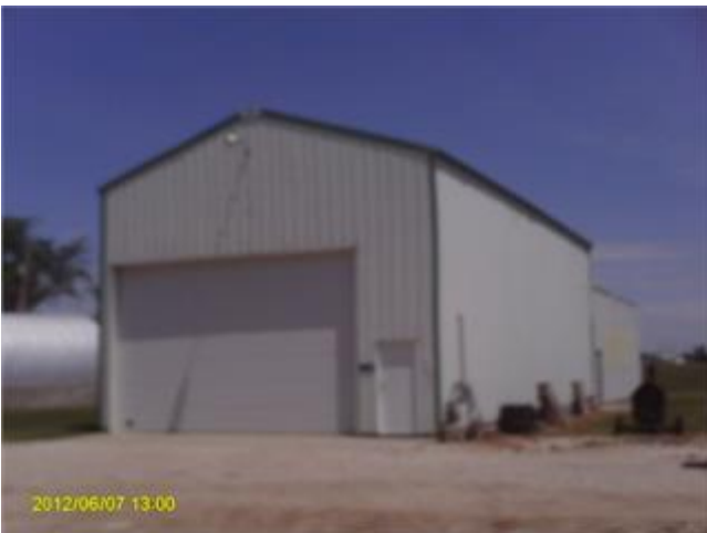
Shop Building - Built 1966, West Portion 30' x 64' Built 2002, East Portion 36' x 48' Doors - 14' High
