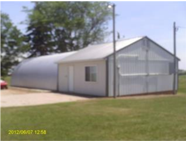
Office Building - Office Area (West) 22' x 24' Storage Area (East) 25' x 44' Built - 1966
