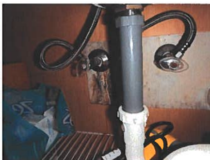
Mold growth and multiple damaged drywall at plumbing.
