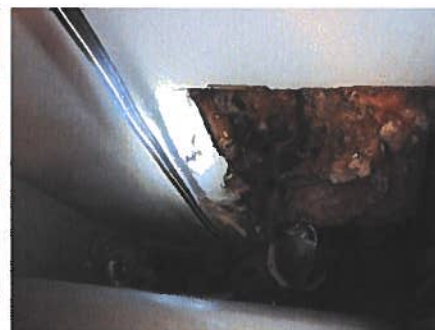
Mold growth and multiple damaged drywall at plumbing.
