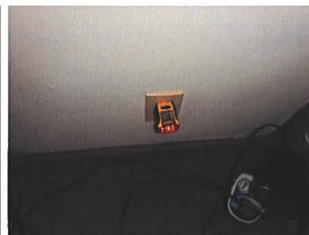
Multiple improperly wired outlets.
