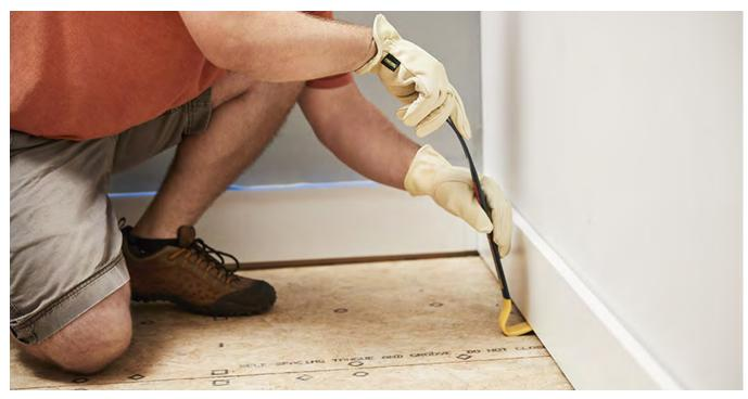
First, remove any baseboards and moldings using a hammer and pry bar.
