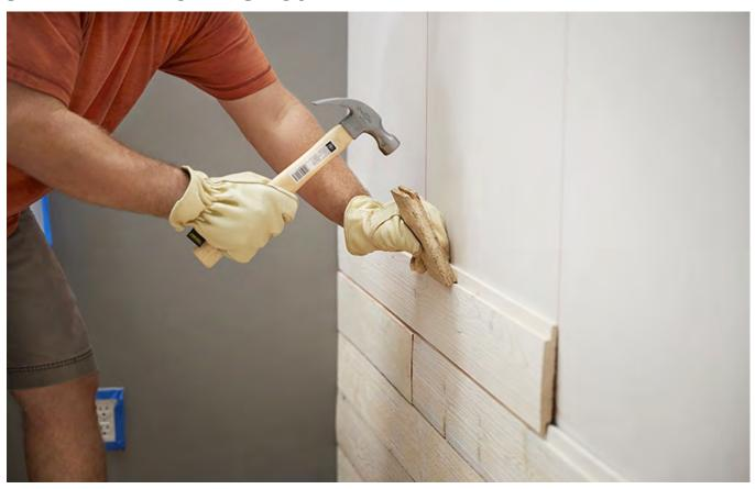
To ensure everything's fitting together tightly, gently tap the shiplap into place before fastening it to the wall.
