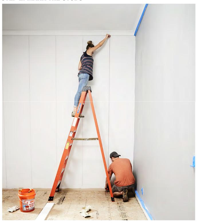
Next, use a stud finder to mark your stud locations on the wall with a pencil, then snap a chalk line along the studs as a guide. While you're at it, measure the wall so you can adjust your layout if the wall is neither level nor square.
