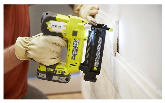
Start at the bottom, and make sure your first **board** is totally **level** before tacking it into place. **Nail** into the groove portion, then add another **nail** into the board itself, making sure to hit studs. Work your way across the room, left to right.
