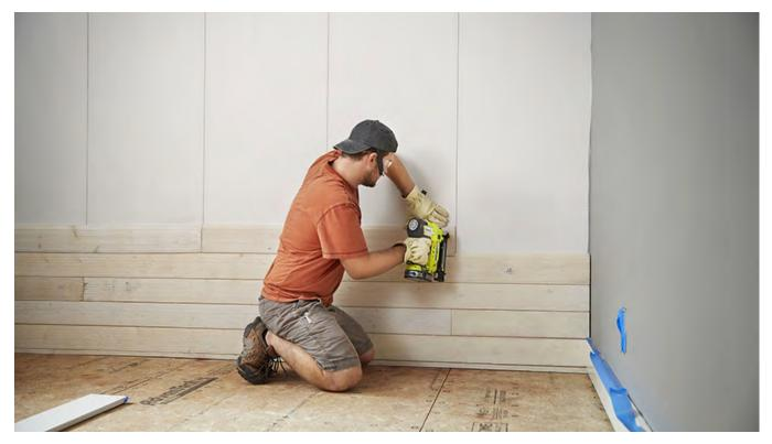
NOTE: Consider the layout as you begin each run. Use a **circular saw** to make each cut. Cut your boards to ensure you land on a stud but also work to achieve a staggered effect running left to right. Also try not to cut any boards shorter than 10-inches wide.
