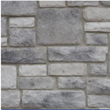
Fireplace Masonry: Buckingham Limestone
