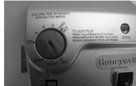
Gas Control shown in the “OFF” position
