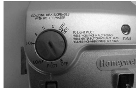
Gas Control shown in the "OFF" position
