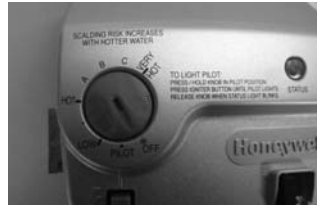
Gas Control shown in the "OFF" position
