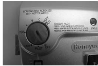
Gas Control shown in the "OFF" position
