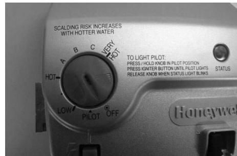
Gas Control shown in the "OFF" position
