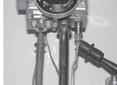
Step 3. If continuity is indicated, the ECO is OK. If continuity is not indicated, the ECO has opened and the combination thermostat/gas valve must be replaced.
