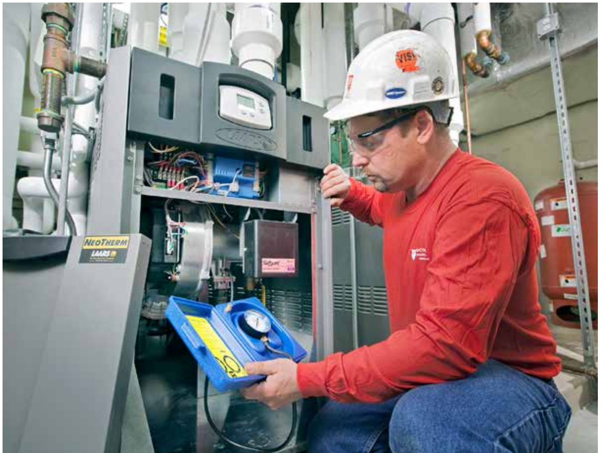
JUST ADD ONE: If total replacement is not an option and a building’s boilers are still in good shape, then adding even one modulating condensing boiler can help reduce operating expenses over time. PHOTO COURTESY OF LAARS HEATING SYSTEMS
