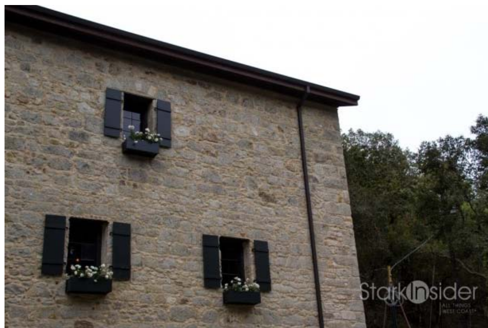
Buena Vista Winery: The exterior of the newly renovated Champagne Cellars.
