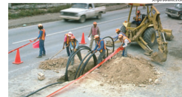
Construction workers unwind a long, hollow strand of shielding through which a fiber-optic cable will be threaded.
