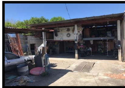
VISTA EXTERNA GALERON (TALLER)
