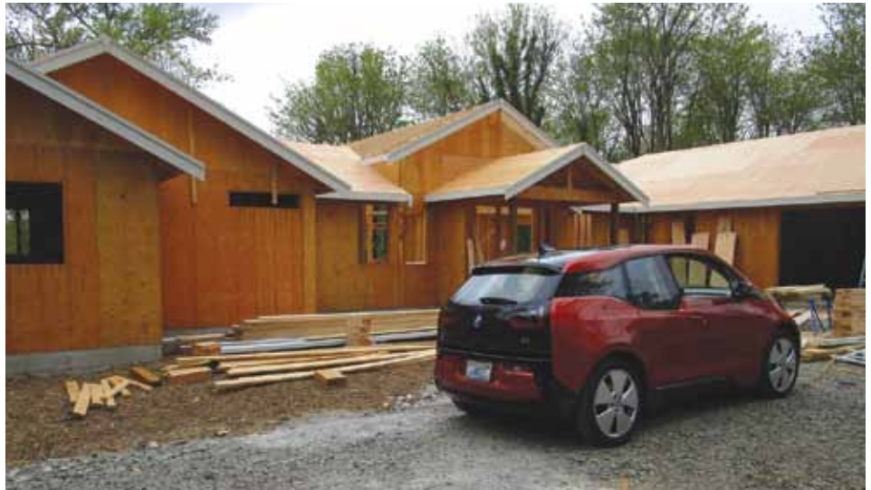
Making the job site rounds.
