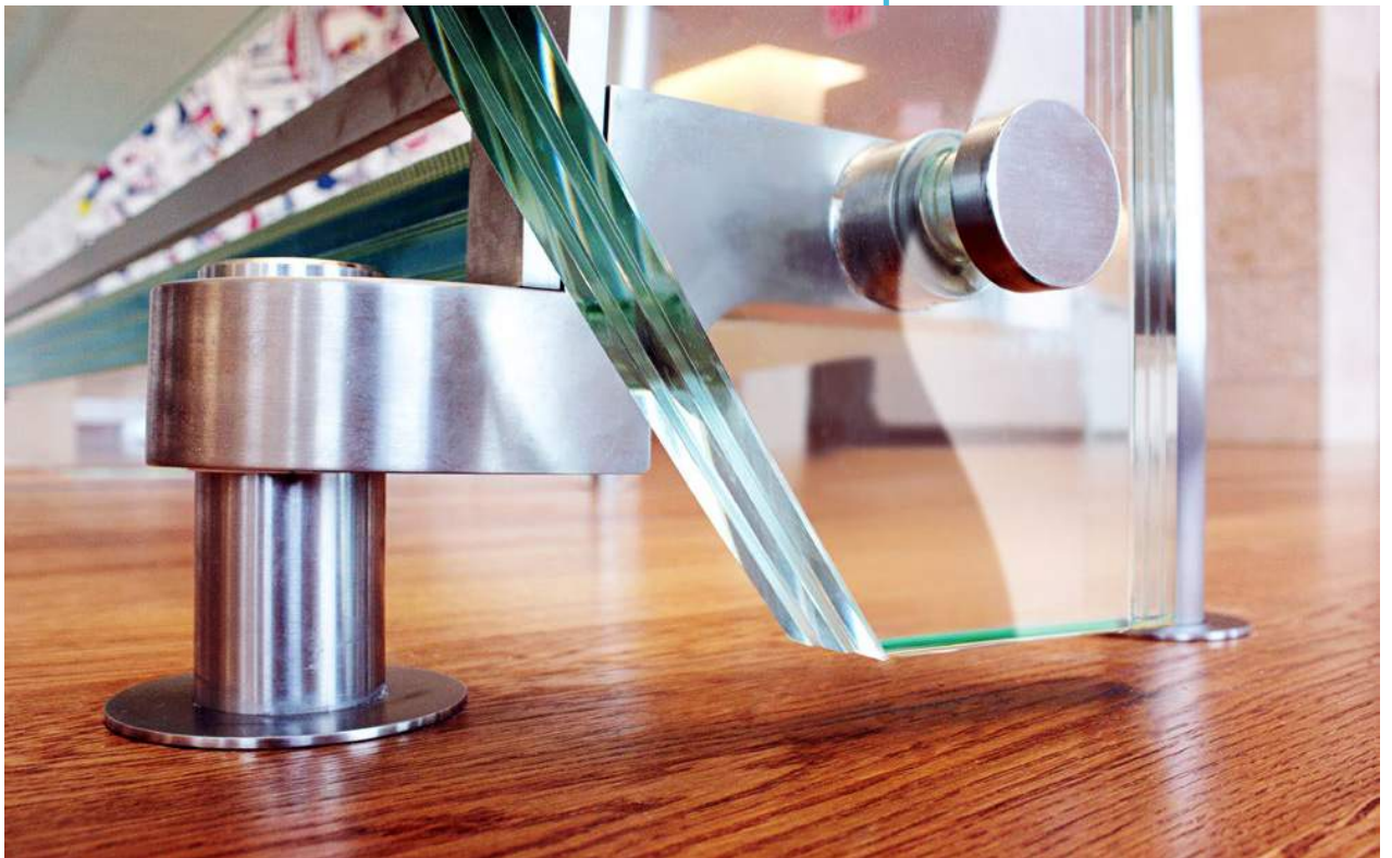
Spiral staircase of structural glass without base support.
