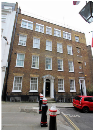
Fig. 42 36 St Andrew's Hill Grade II | Late C18
