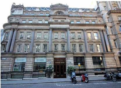
Fig. 48 Finsbury House Grade II | Late C19
