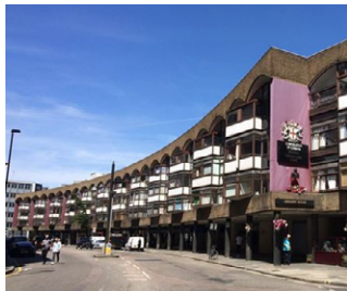
Fig. 62 Crescent House Grade II* | Mid C20
