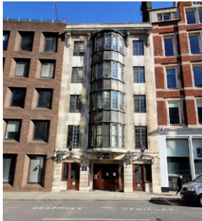
Fig. 34 Snowhill Police Station Grade II | Early C20
