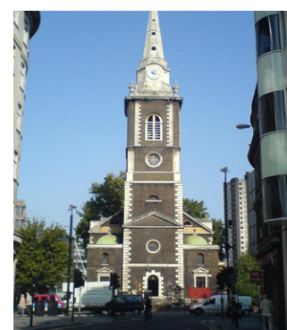
Fig. 21 St Botolph's Algate Grade I | Mid C18
