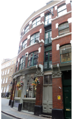
Fig. 59 31-32 St Andrew's Hill Grade II | Late C19
