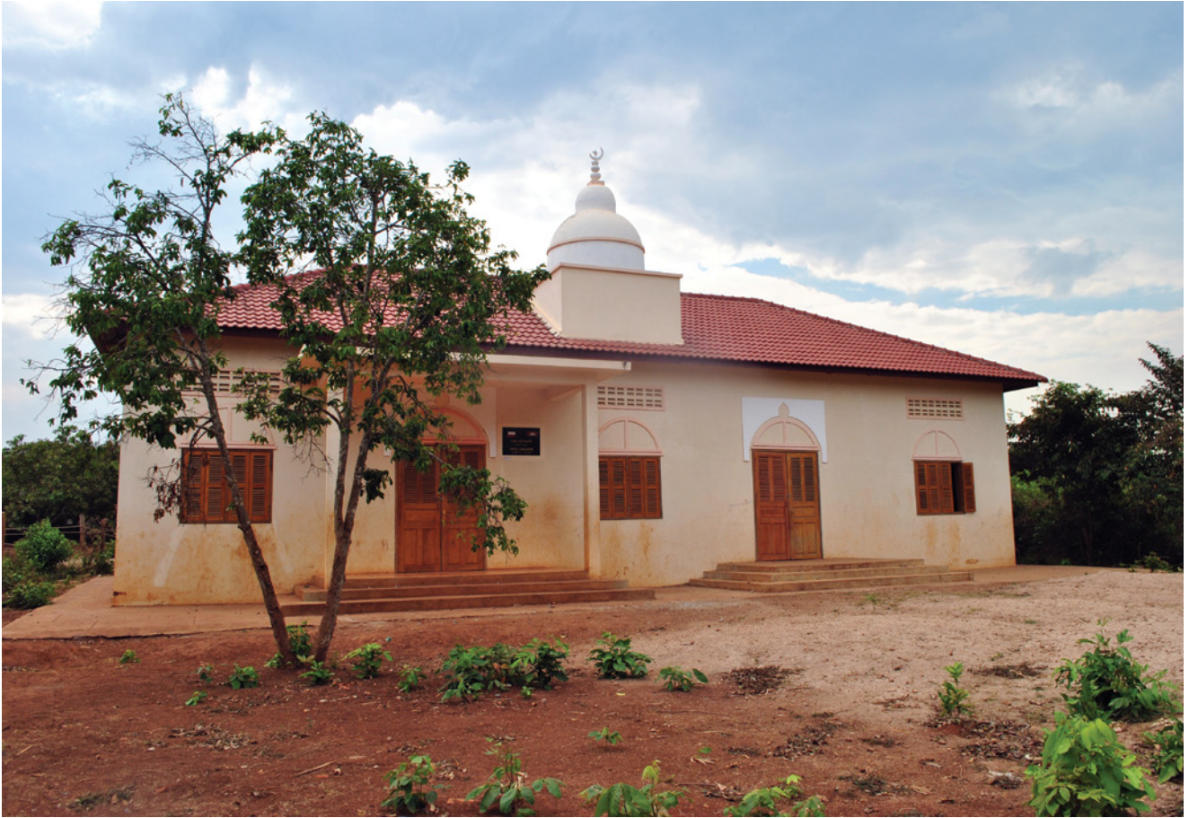
□ Figure 3: New Kuwaiti-funded Mosque near Lae Village
