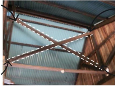
Kahoy na Cross Bracing
