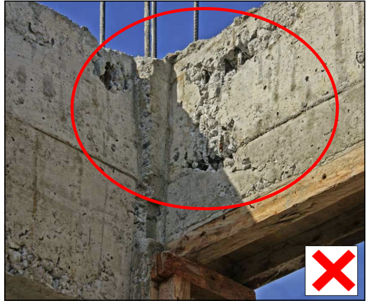
With small holes and exposed rebars.
