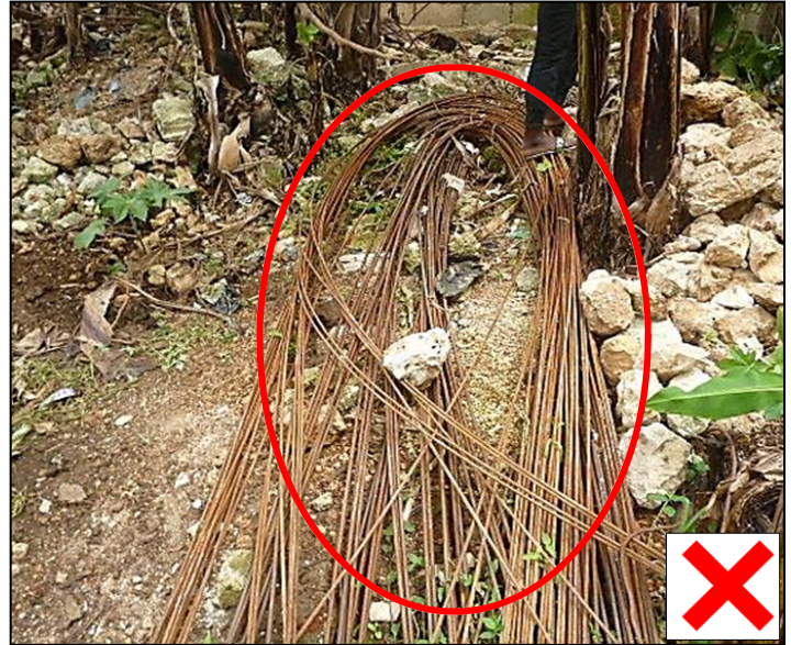
Exposed to rain and bent bars.
