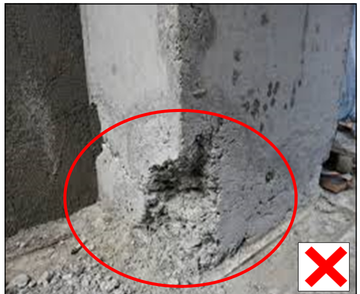
With small holes and exposed rebars.
