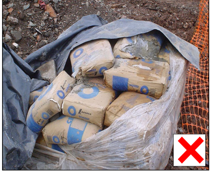
Wet and open or broken bags.
