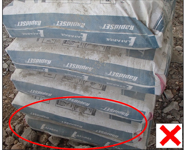
Piled directly on the ground.
