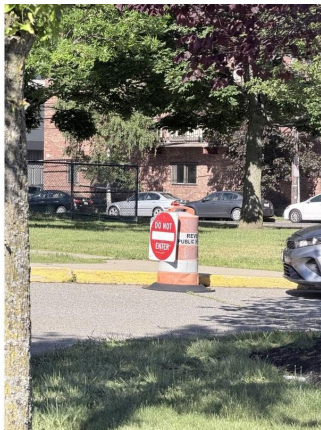
Close view of the temporary do not enter control.
