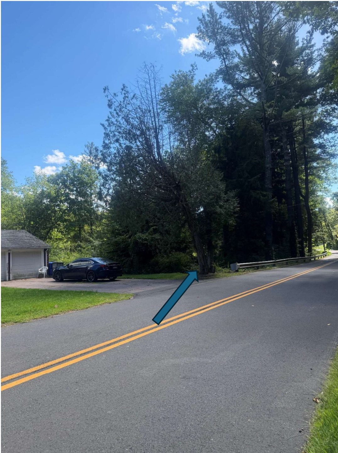
Area 4 – dying arborvitae near driveway/culvert
