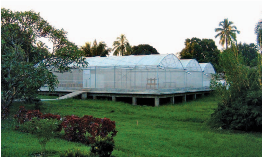
FIG. 2. Modular mosquito containment facility at the Ifakara Health Research and Development Centre in Tanzania. (Photo courtesy of Dr. Michael Gottlieb.)
