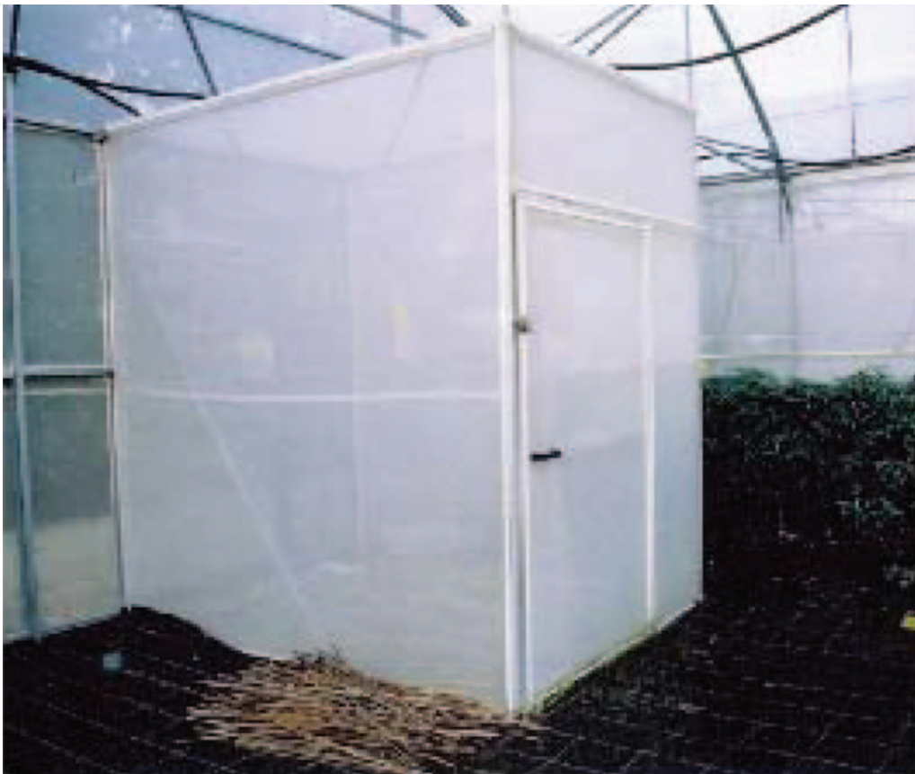
FIG. 3. A containment vestibule for entry into individual cages to enhance protection against escape. (Photo courtesy of Dr. Bart Knols.)
