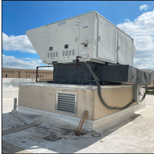
Figure 5: Roof system at the Sleep Inn
