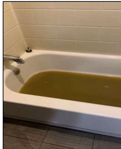
Figure 2: Tub drain backing up
