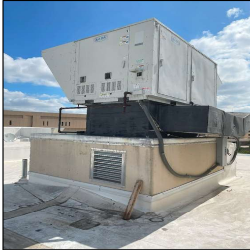
Figure 5: Roof system at the Sleep Inn
