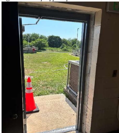
Figure 8: Door propped open due to chemical smell
