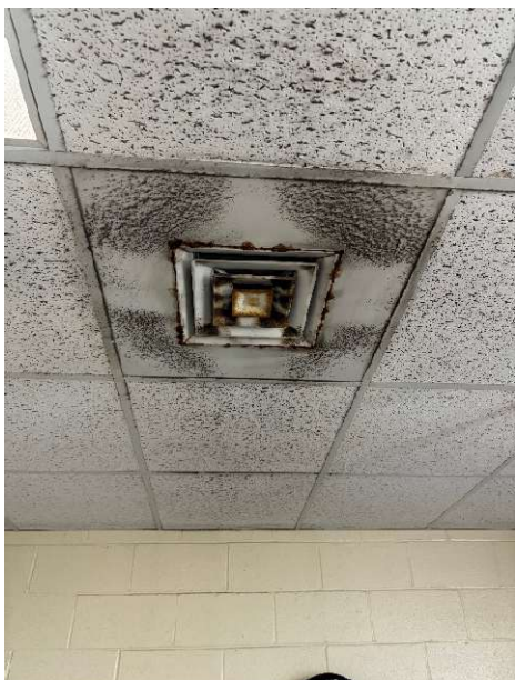
Figures 12&13: Unknown black particulate matter on vents
