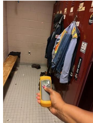
Figure 3. Temperature on wall across from AC unit
