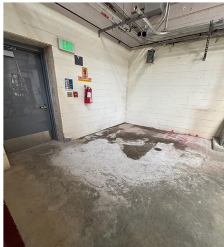
Figure 1. Floor repair at entrance to RSPS 2
