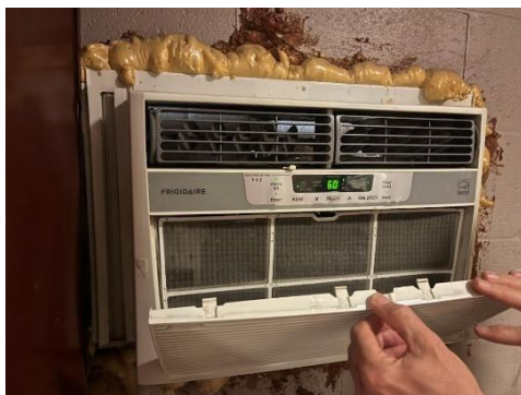
Figure 4. AC Filter free of debris
