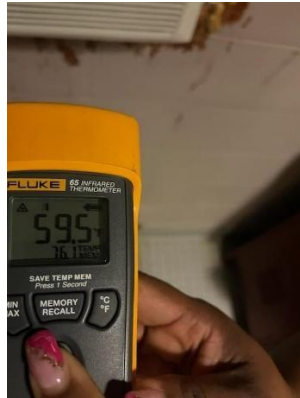
Figure 2. Temperature on AC discharge
