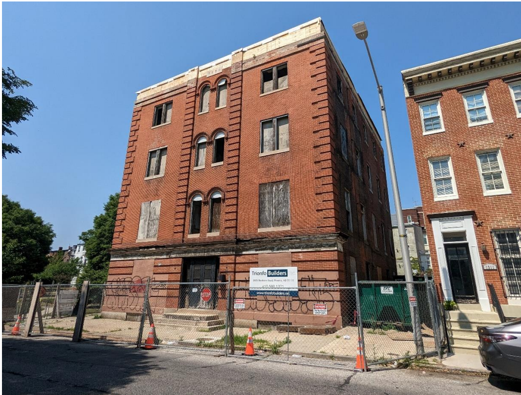
Image 19: Façade and east elevation.
