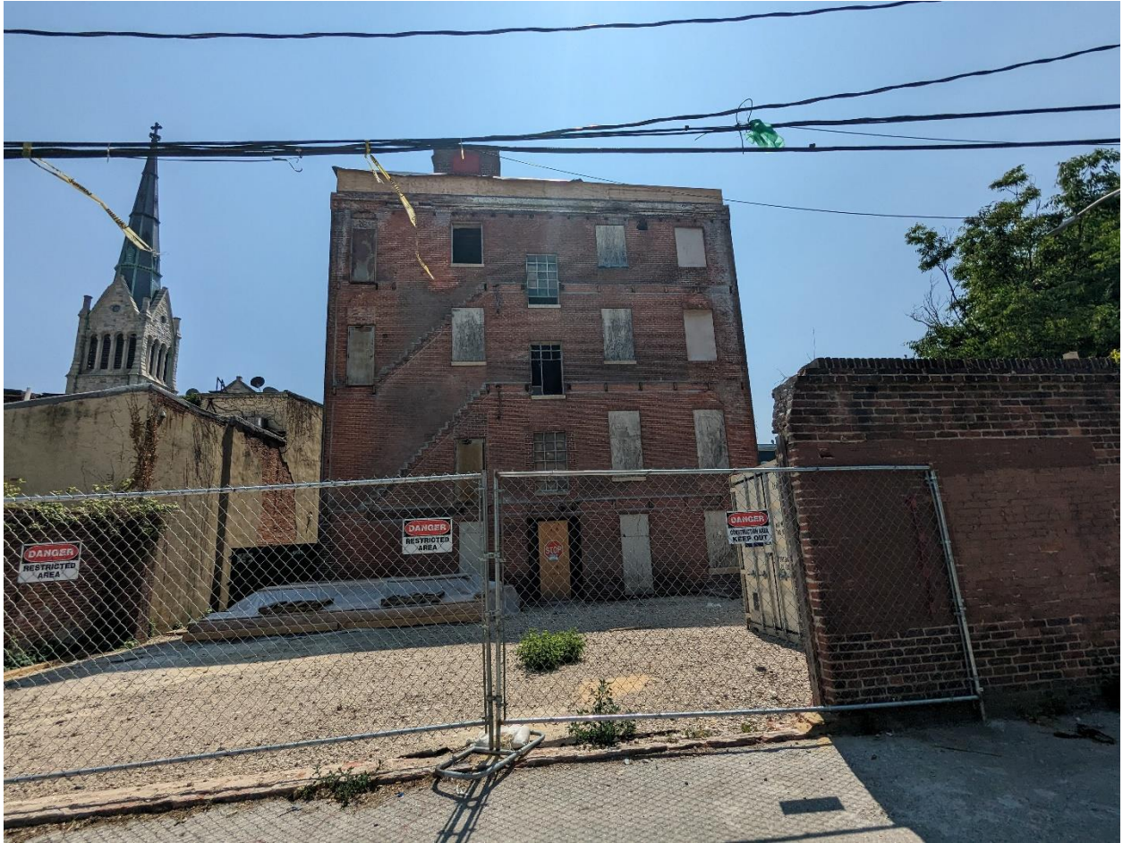
Image 22: Rear elevation, viewed from Stoddard Alley.
