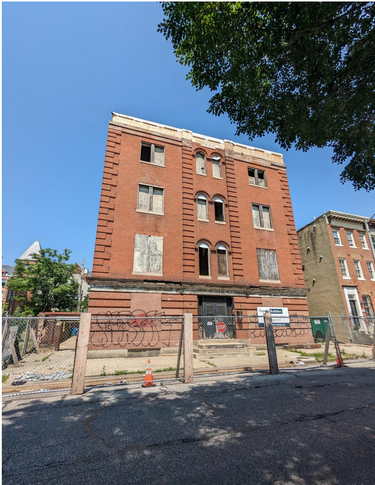
Image 18: Façade, facing Druid Hill Ave.
